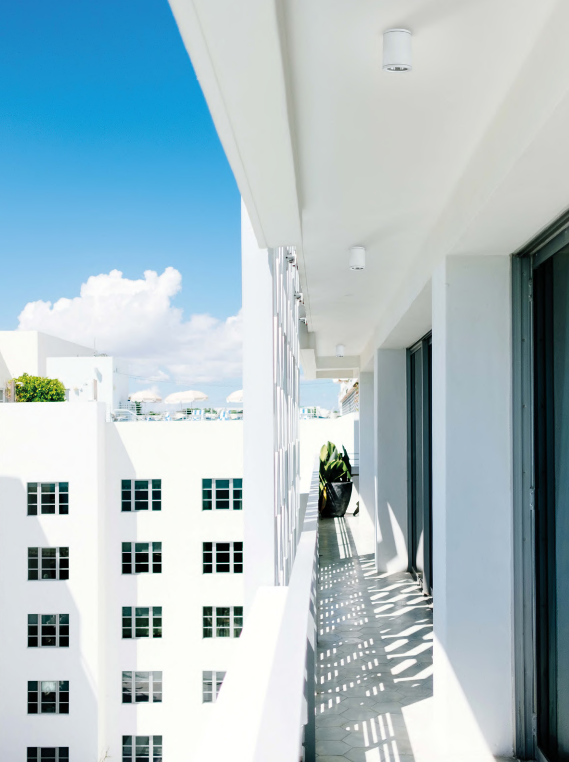
OUTDOOR - CEILING FIXTURES
